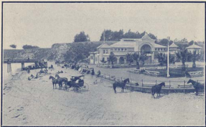
NEW BATH HOUSE, SANTA BARBARA
