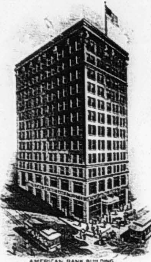
AMERICAN BANK BUILDING
