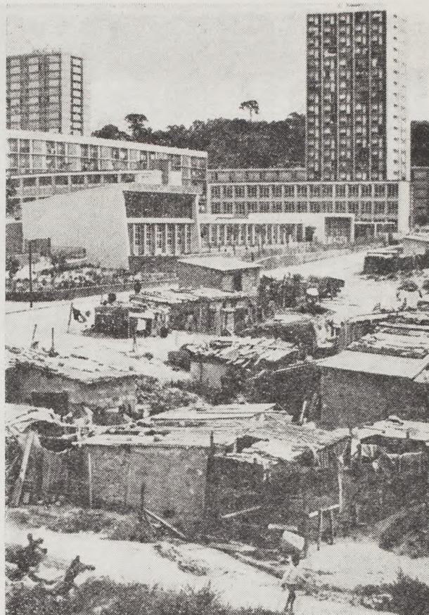
Contrast under the capitalist regime. Alongside modern blocks of flats are to be found shanty-towns and slums for immigrants. (ILO photograph)
