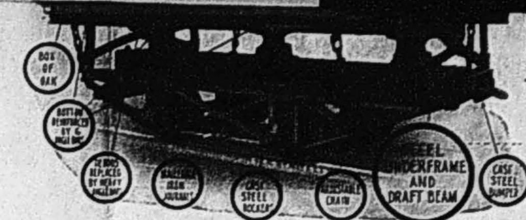
Fig. 12349—4 yd. Square Box Dump Car.
