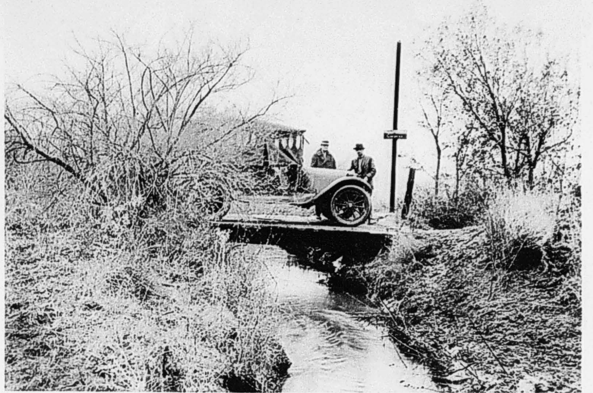
Fig. 1. Escondido Mutual Water Company's Supply Ditch.
