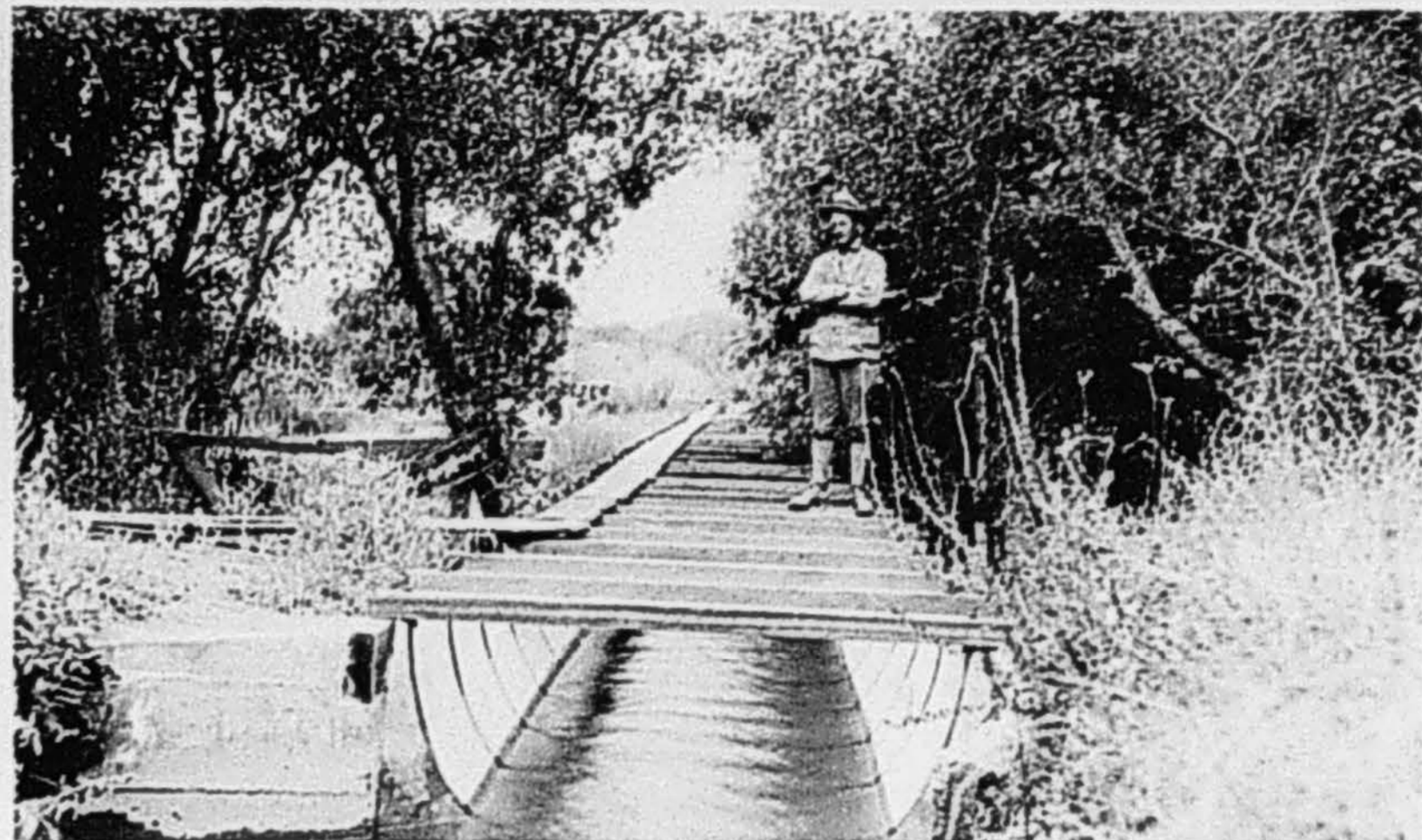
Fig. 1. Metal Flume Section, Escondido Mutual Water Company's Supply Conduit.
