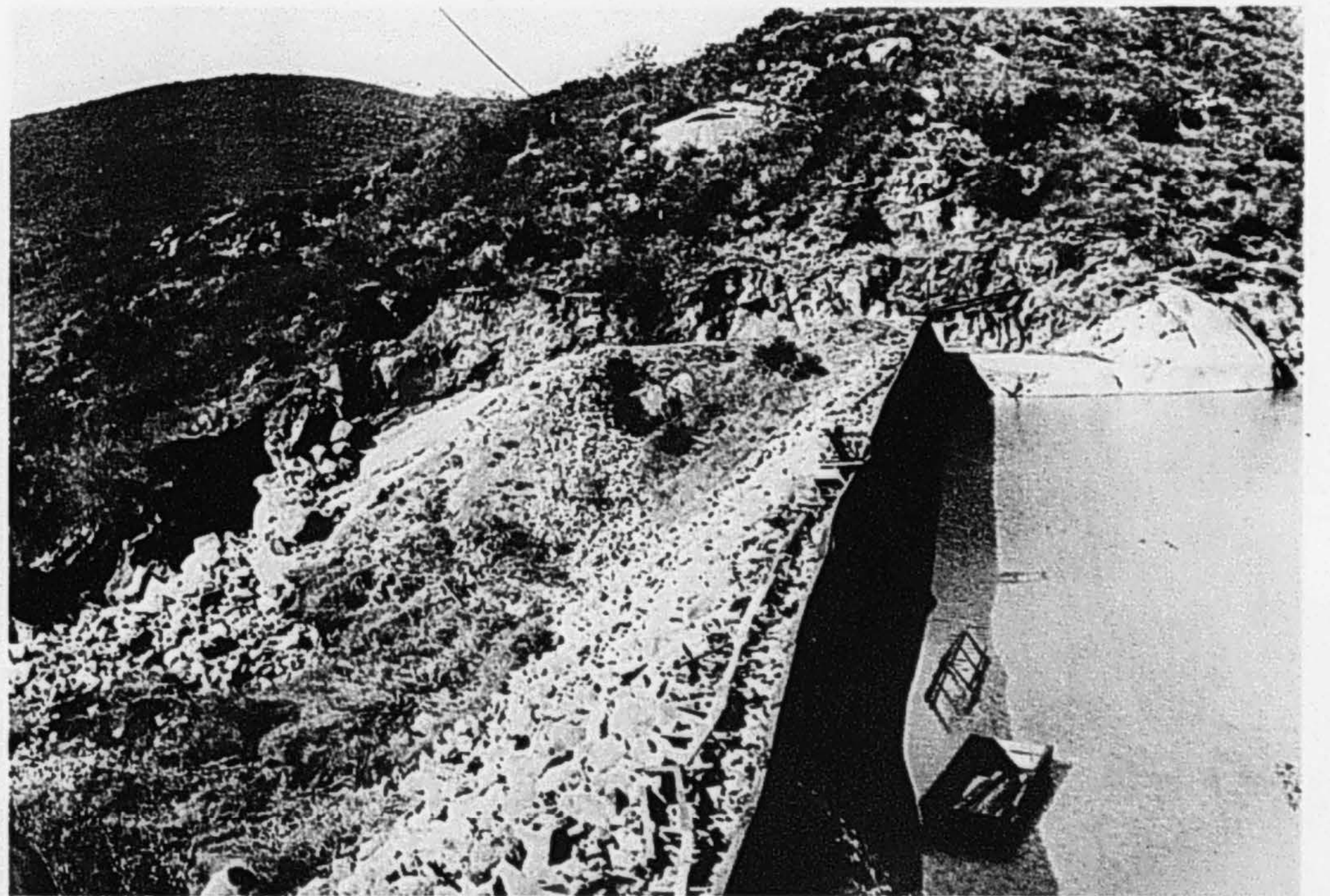
Fig. 2. Storage Dam, Escondido Mutual Water Company's Bear Valley Reservoir.
