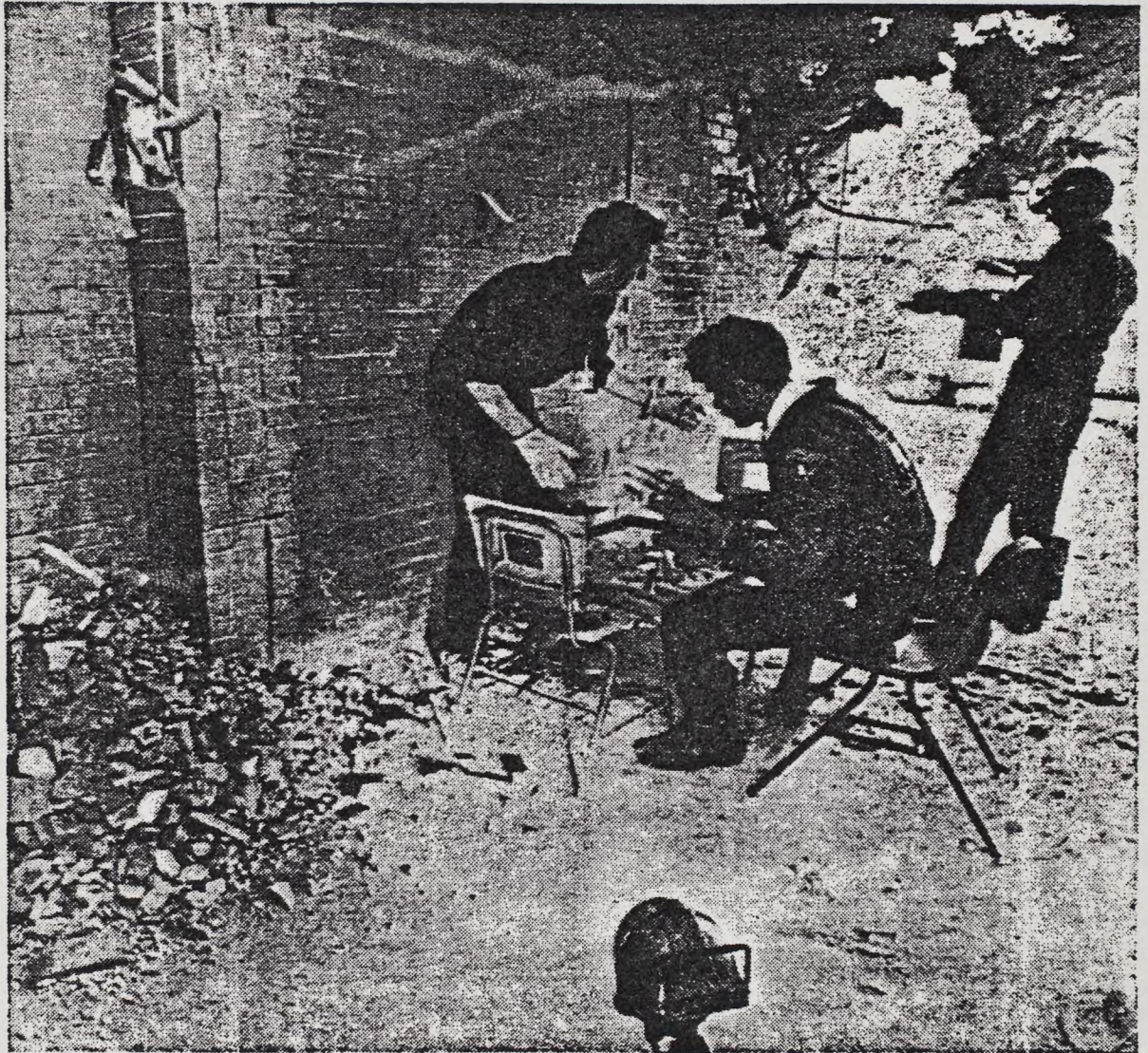
BOMB DAMAGE — Cleveland police sift through the rubble of the Martin Luther King Jr. Vocational High School where a bomb exploded early Wednesday causing extensive damage. The
